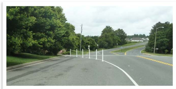
Flexible bollards were installed on Mill Road to discourage motorists traveling southbound on Mill Road from passing drivers in a parking lane (looking north)
