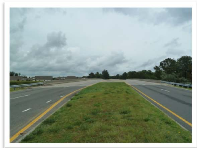
Mill Road overpass over Interstate 295 (looking north)
