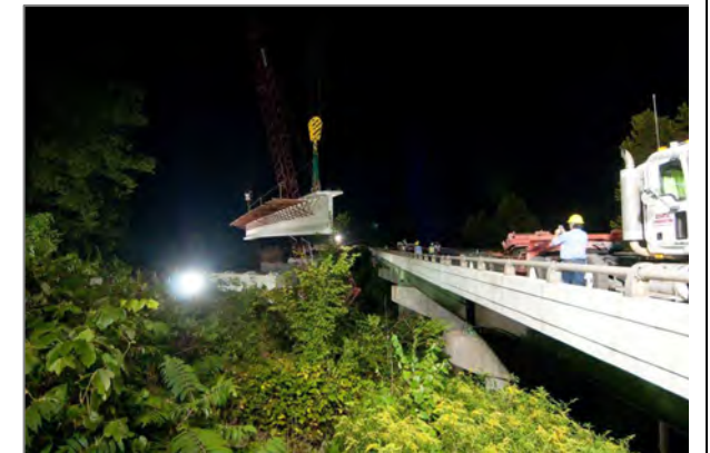
Setting bridge beams at night.
