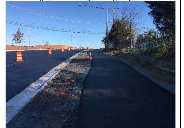
Road widening and bicycle lane
