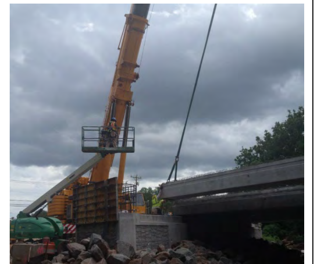
Placing of box beams for bridge replacement
