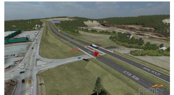
US 219 Bridge over US 40 Alt.
