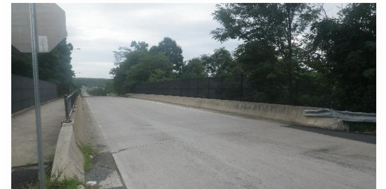
Existing Backlick Road Bridge (looking South)
