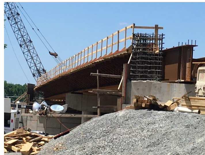
Two-span steel plate girder with semi-integral abutments
