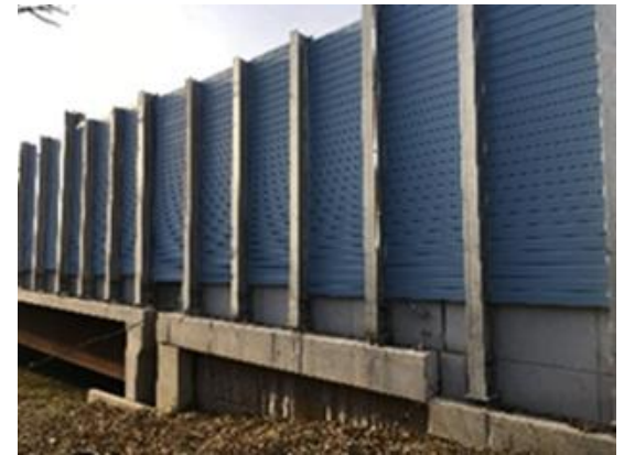
I-95/I-395 (THN Ramp) – Lightweight Noise Wall Barrier on Bridge
