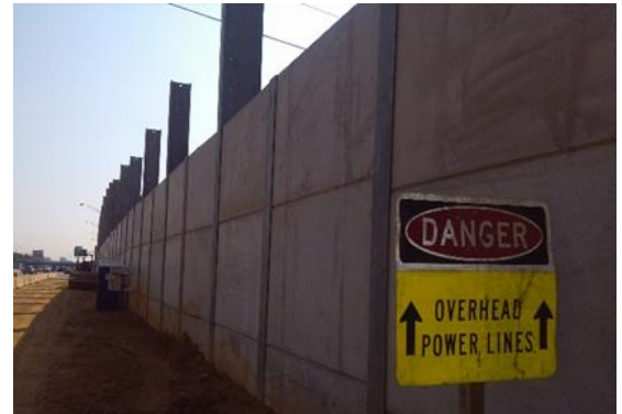
I-95/I-395 (THN Ramp) Noise/Retaining Wall Combination Walls
